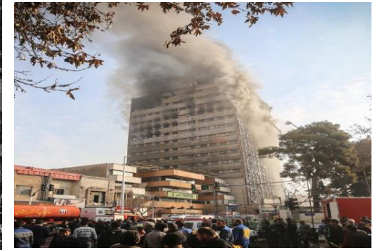
Building fire and collapse
